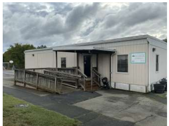
36 - JUDY CENTER MODULAR BUILDING
